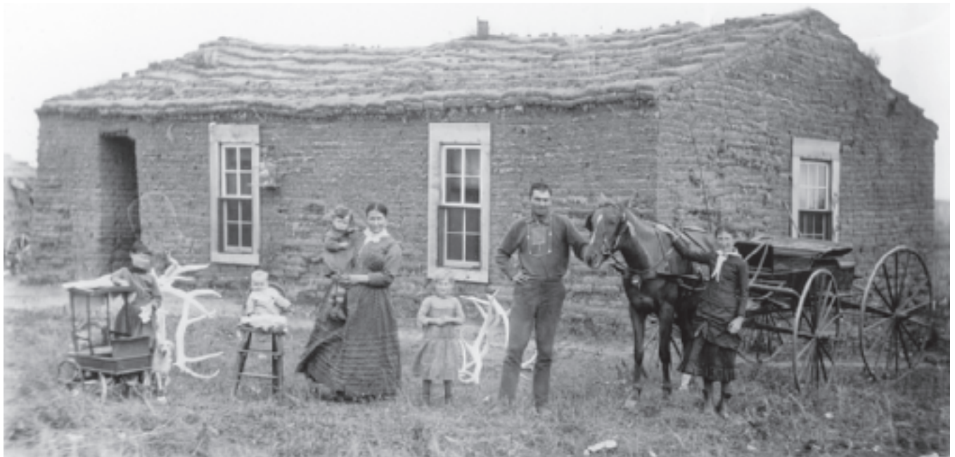
SODBUSTERS As farmers moved onto the Great Plains in Nebraska and other states on the agrarian frontier, their first task was to cut through the sod that covered the land to get to soil in which they could plant crops. The sod itself was so thick and solid that some settlers (including the Summers family of West Custer County, Nebraska, pictured here in 1888) used it to build their houses. The removal of the sod made cultivation of the plains possible; it also removed the soil's protective covering and contributed to the great dust storms that plagued the region in times of drought. ( Nebraska State Historical Society )
